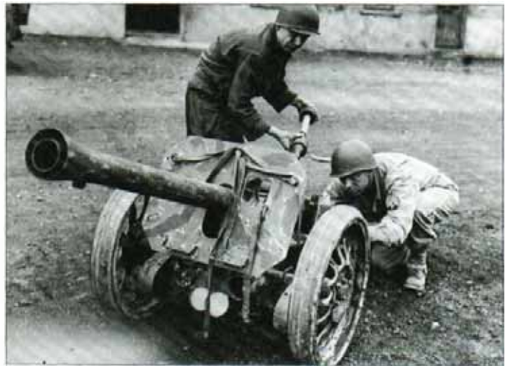
The 8.8-cm (3.46-in) Raketenwerfer 43 or 'Puppchen' was a form of anti-tank rocket launcher that was superseded almost as soon as it entered service in 1943 by the RP 43 series firing a very similar rocket. The RP 43 could be produced far more cheaply and quickly than the Puppchen, here being examined by Americans.
