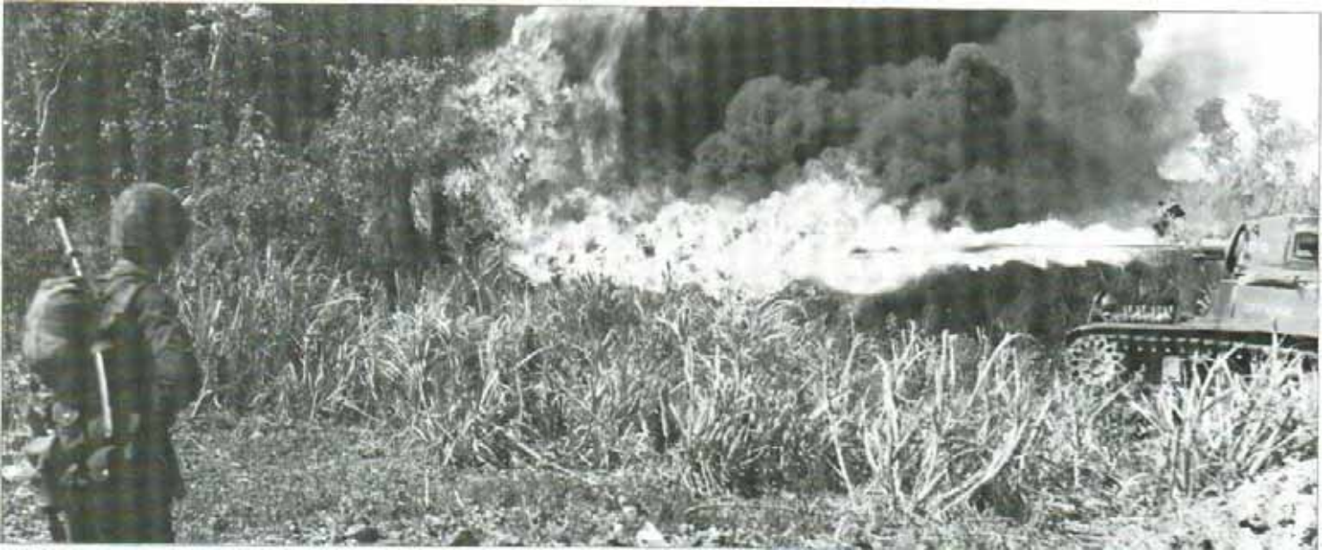
Below: The Sherman Crocodile was a British development to use Shermans in the flame-throwing role, but only four were ever produced as US Army interest in the project waned almost as soon as it started. The flame gun was mounted to the right of the hull gunner's escape hatch.
