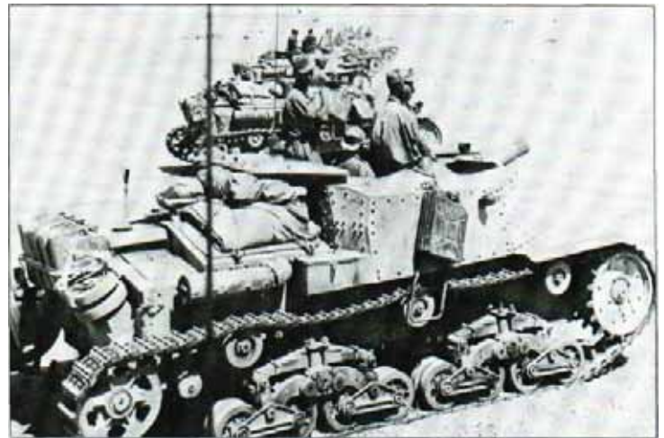
Above; M13/40s in the desert, 1941. These are the Semovente Comando version, without turrets and with additional radio gear. Many were abandoned by the Italians and taken over by the British.
