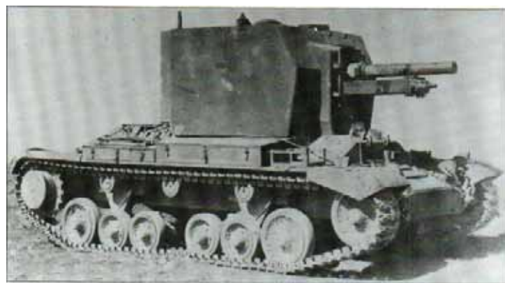
Above: This Bishop in 'factory's taste' clearly shows the high and bulky outline of the fixed turret mounting the 25-pdr gun. As this was a 'first
