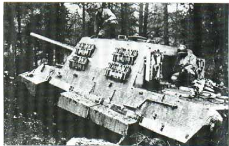
Above: Two types of suspension were used on the Jagdtiger. This example has the Henschel suspension; the other type used larger road wheels from Porsche. Based on the Tiger II tank chassis, only about 70 were produced, and it was the heaviest AFV to see service during World War II.
