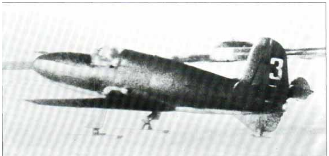
Above: The third prototype BI was fitted with retractable skis which could be interchanged with wheels depending on the ground conditions. Armament was two 20-mm cannon.
