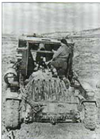
Above: A Bishop on the ranges with the gun detachment commander outside the fixed turret, as there was room for only two gunners inside. The fixed turret restricted the barrel elevation and thus range.
