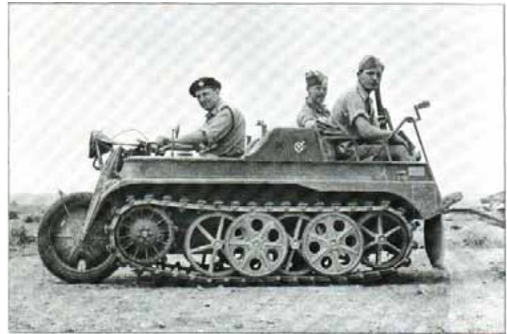
British soldiers try out a captured SdKfz 2 kleines Kettenrad. The driver sits in a well between the two tracks, with the engine just behind him.
